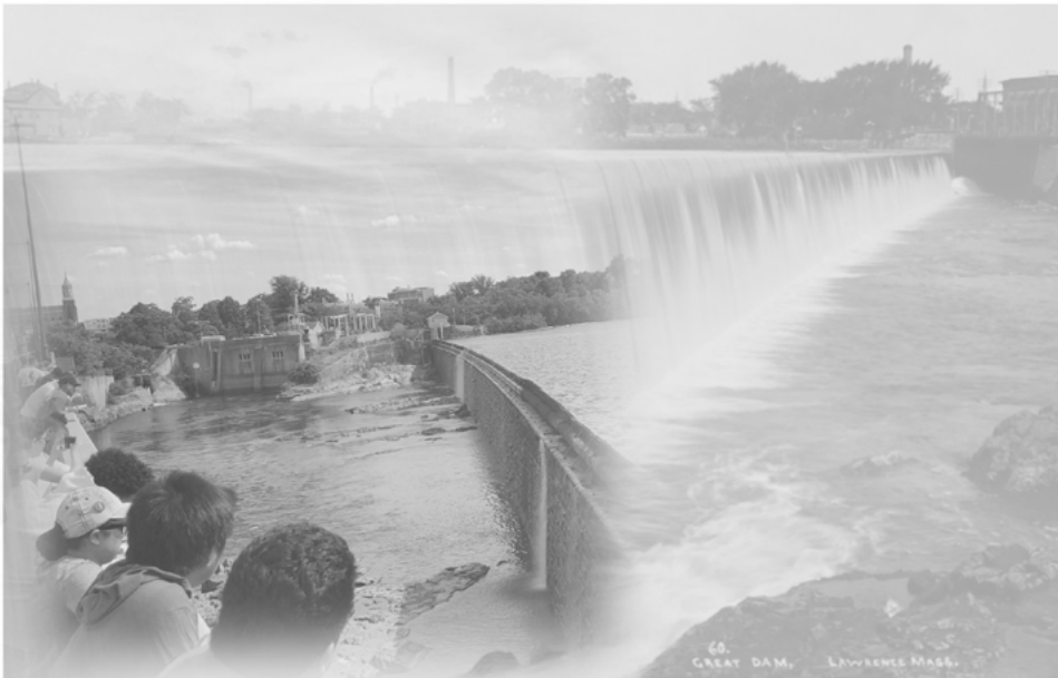
Figure 4: Lawrence Great Stone Dam, Lawrence. Source: Lawrence History Center, Accession 2003_012_004; and (left) Station1 Fellows visiting and learning about the Great Stone Dam in 2019 as part of the curriculum on socially-directed science and technology. Source: Station1, 2019.
